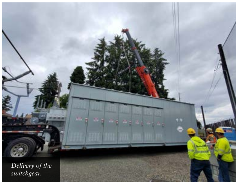
Setting the transformer.
